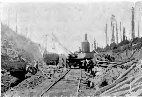
JACOBY CREEK QUARRY — LOCOMOTIVE CRANE SWITCHING CAR THROUGH THE AIR.
